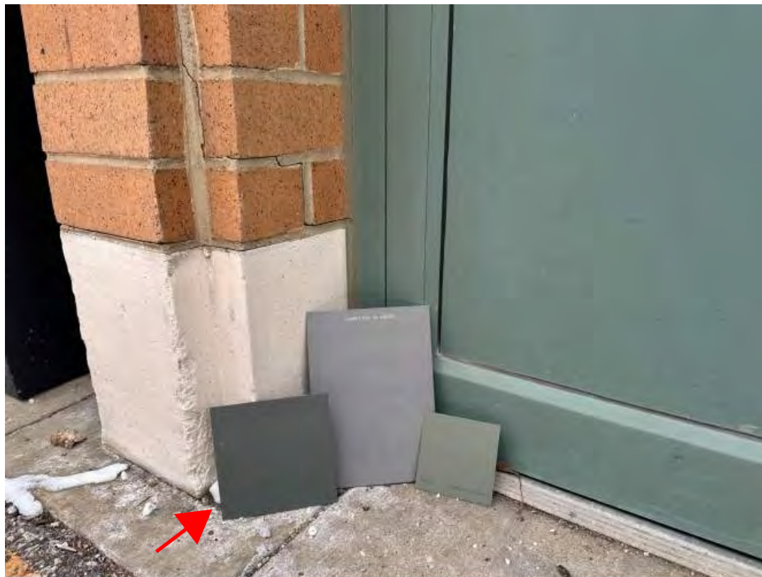
ARCADE | BRICK, BASE AND EXISTING GARAGE DOOR
