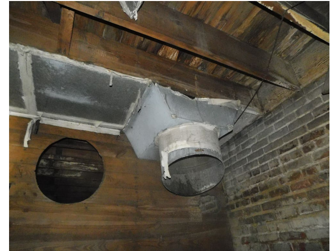
Ducts with asbestos
