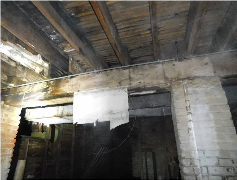
Thermal System Insulation (TSI) asbestos scrap
