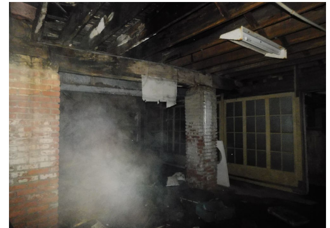
Ducts with asbestos
